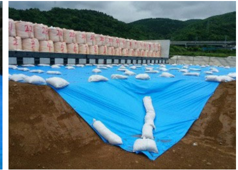
Sample countermeasure against rain
