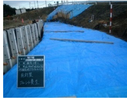
Sample countermeasure against rain
