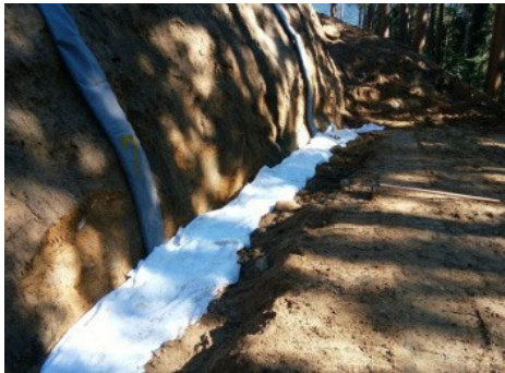
Sample drainage of cut and fill boundary area
