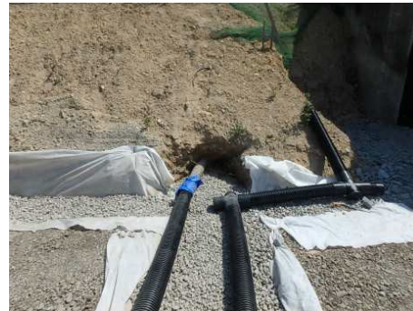
Sample countermeasure against spring water
