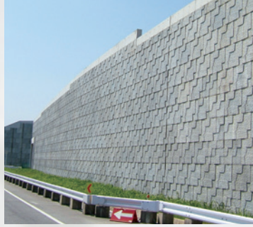
Materials for reinforced soil method
