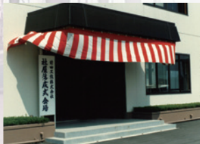
Harue Headquarter office and factory newly built
