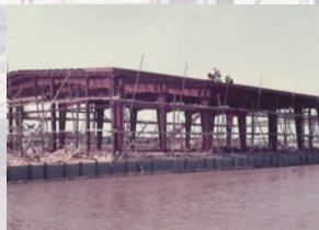
Headquarter office and factory newly established
